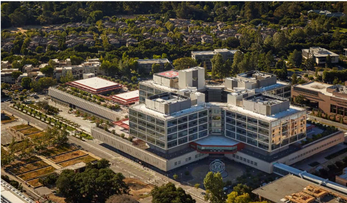
Aerial photo of the new Stanford Hospital—photo courtesy of Stanford Health Care
