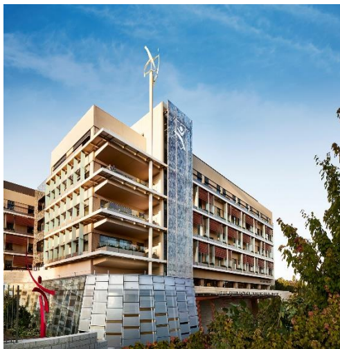
Photo rendering of Lucile Salter Packard Children’s Hospital at Stanford’s expansion project at its main hospital, partially financed by CHFFA Series 2022 A bond proceeds
