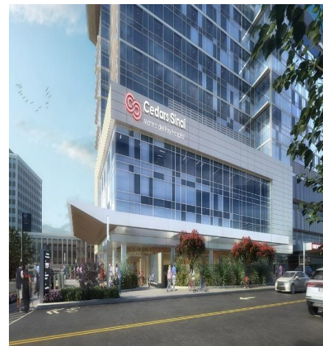
Photo rendering of Cedars-Sinai Health System’s replacement hospital in Marina Del Rey, partially financed by CHFFA Series 2021 A bond proceeds
