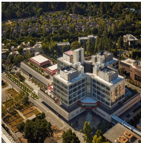
Photo rendering of Stanford Health Care’s new Stanford Hospital, partially financed by CHFFA Series 2021 A bond proceeds
