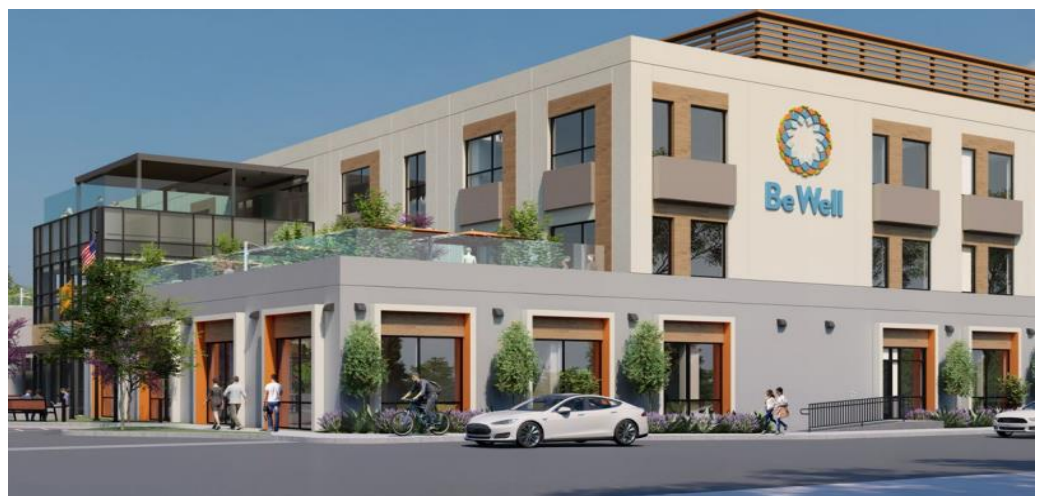
With programs within the building partially financed by a grant award from CHFFA, Orange County's Be Well Orange Campus provides mental health and substance use treatment services to Orange County residents who are referred for care.
