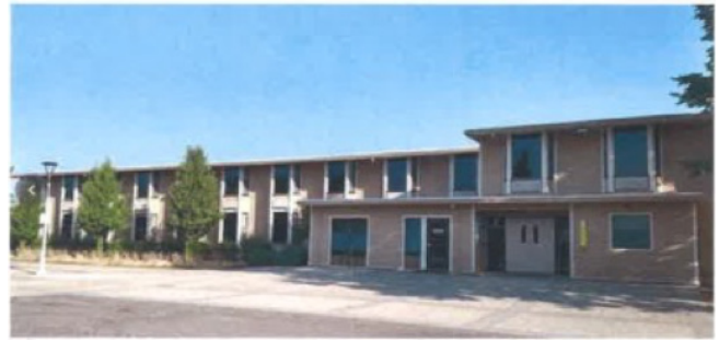
Sierra College is replacing and expanding existing housing.
