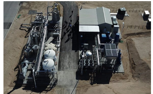
Top picture: CARB-compliant Compressed Natural Gas collection vehicle, Amador Valley Industries, LLC. Bottom picture: SoCal Biomethane, LLC project.
