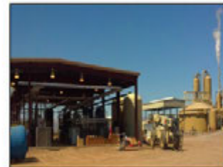
Figure 2: Upgraded and relocated demonstration plant
