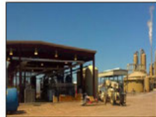
Figure 2: Upgraded and relocated demonstration plant
