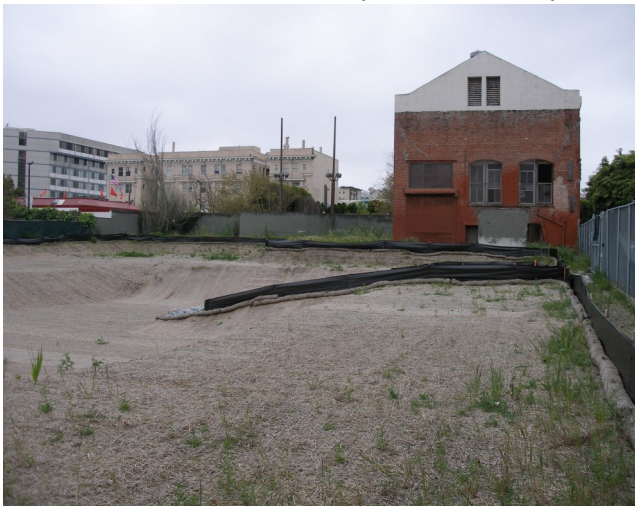
Before: Vacant former railway maintenance yard
