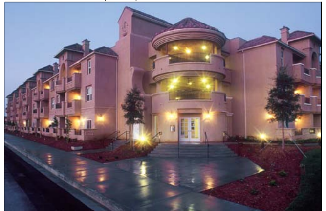
Arbor Gardens (after)
