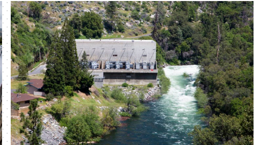
Kirkwood Powerhouse and Penstock
