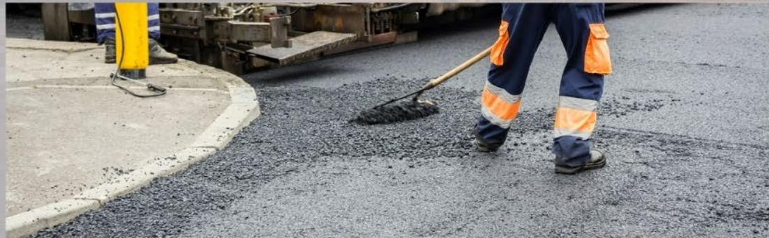
Construction and Maintenance of Streets and Infrastructure
