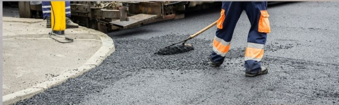
Construction and Maintenance of Streets and Infrastructure
