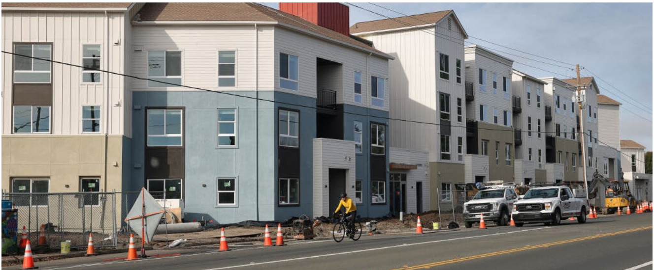
Shiloh Crossing in Windsor opened in December 2024 and offers 134 affordable homes for families earning 30-70% AMI. The project received federal 4% LIHTCs and enhanced state LIHTCs as part of the CalHFA MIP set-aside in 2022.
